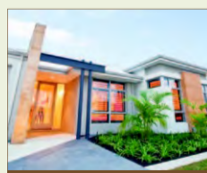
Switch eight 80 Vertu Estate, Harrisdale.
