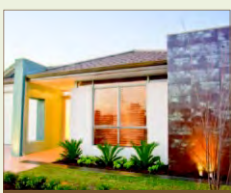
Switch eight 100 Emerald Park, Wellard.
